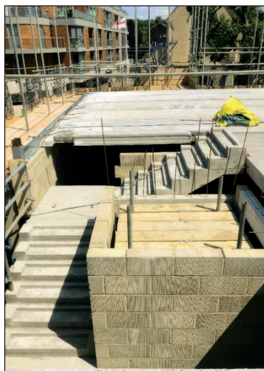
The stairs and lift well
