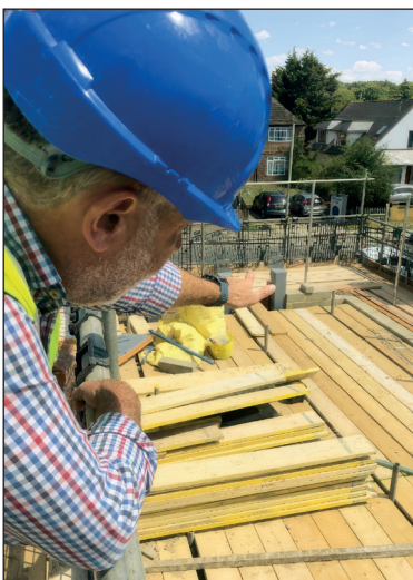
Don, the works manager, above the interior roof of the community chapel
