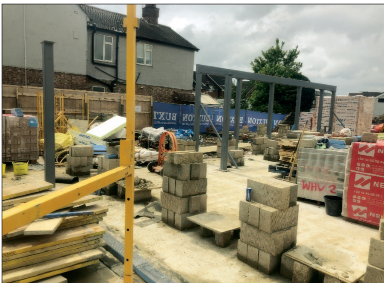
The framework for the walls of the dining room, facing into the courtyard
