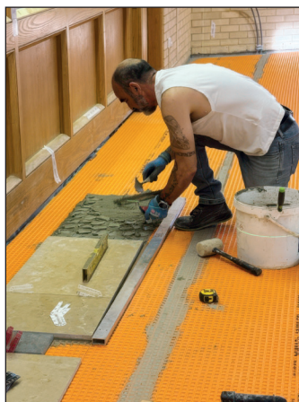
Laying the first tile
