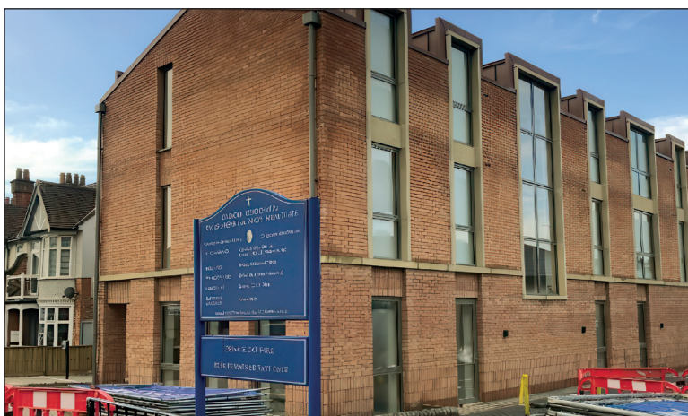
The work almost completed, showing the long window of the stairwell along the side and the windows of the Community Room on the ground floor, to the front of the building
