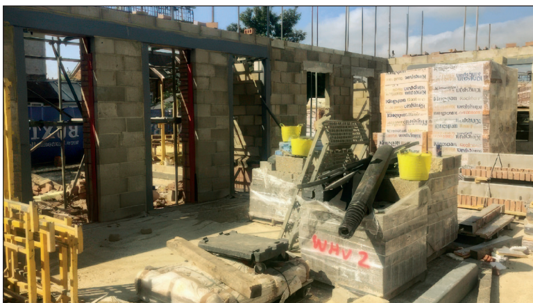
The walls of the future dining room, looking into the courtyard
